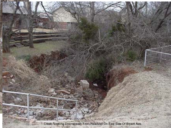
Creek Looking Downstream From Headwall On East Side Of Bryant Ave
